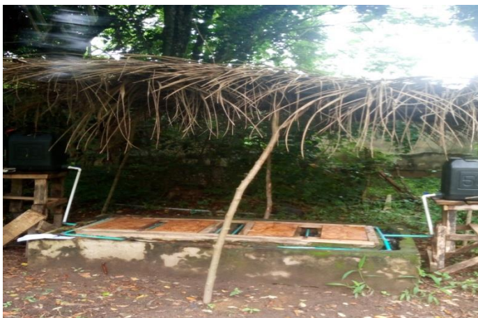
Plate 1: The Refurbished Evaporated Facility With Its Reservoirs, A Pipe Layout And The Shed.
